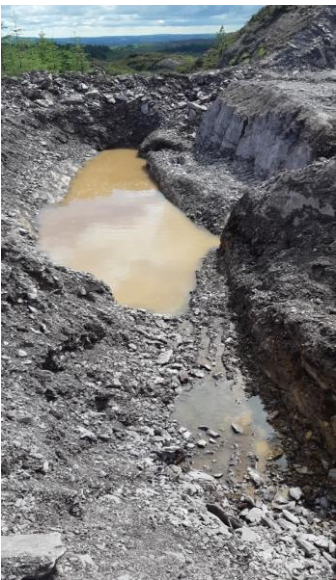
Lower channel before pumping, squared rock profile (RHS), bedrock rising to extreme north (LHS)
