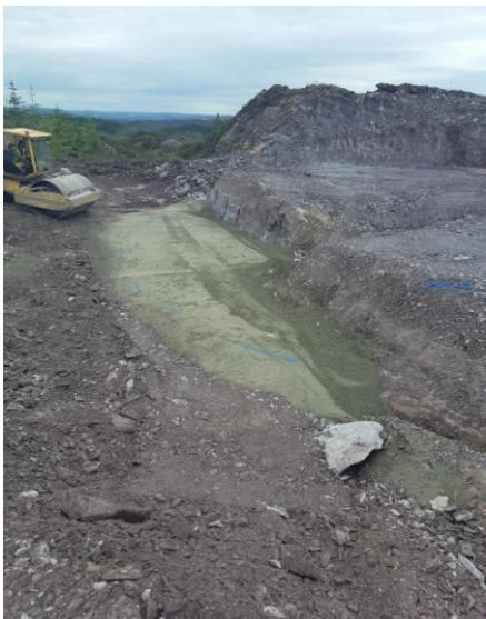
Initial placement of dry leanmix to lower channel
