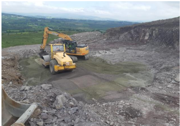
Placement of leanmix on lower tiers to west
