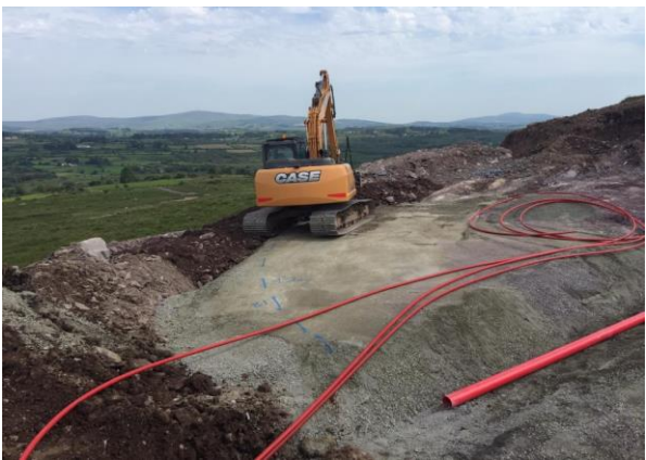
Placement of leanmix infill to northwest
