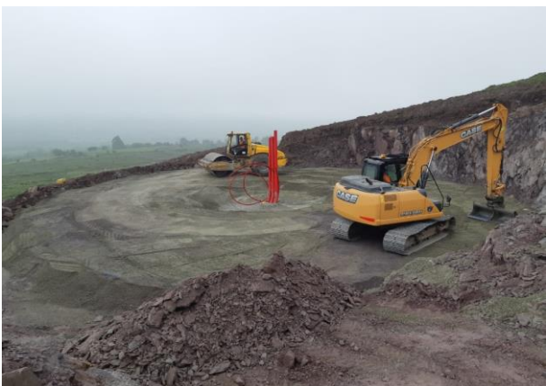
Final blinded formation area being prepared
